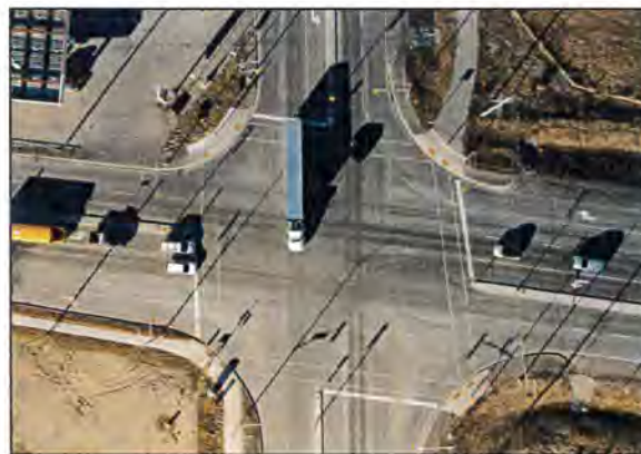
County Capital projects expenditures include a number of road and bridge rehabilitation and construction projects.
