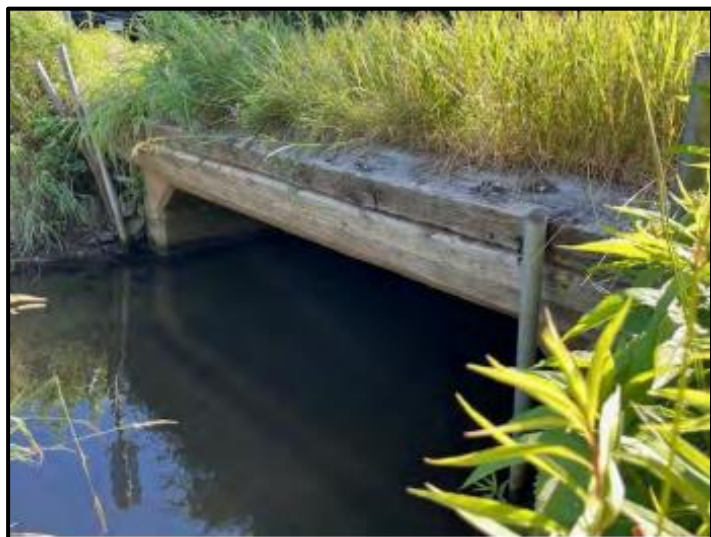
Culvert No. 24 – 8th Line (BCI = 73.2 Good)
