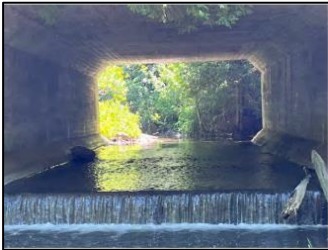
Culvert No. 14 – 5th Line (BCI = 60 Good)
