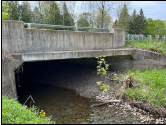
Culvert No. 14 – 5th Line (BCI = 60 Good)
