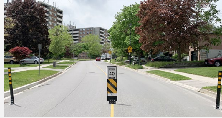
Centreline Bollards / Flex Bollards
