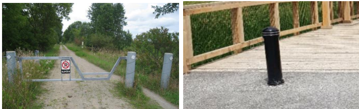
Figure 12: Photos (left to right) Swing Gate (P-Gate), Bollard (Permanent or Removeable)
