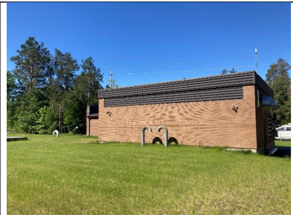
FIGURE 2 - EXTERIOR OF MILL STREET (EAST) SITE
