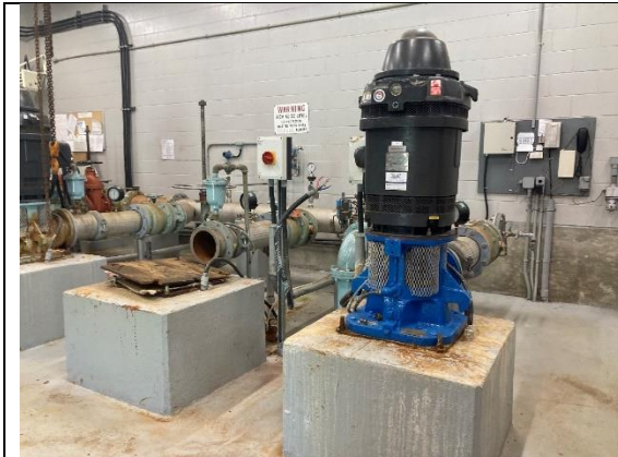
FIGURE 5 - INTERIOR OF EXISTING MILL STREET PUMPHOUSE (EAST) SITE
