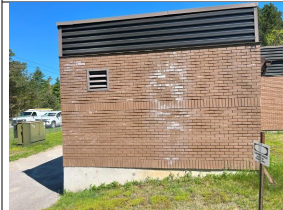
FIGURE 3 - EXTERIOR OF MILL STREET (SOUTH) SITE
