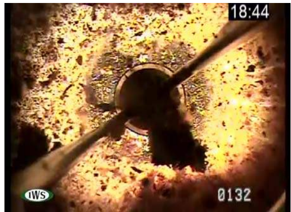
Approaching well bottom at 132 feet
