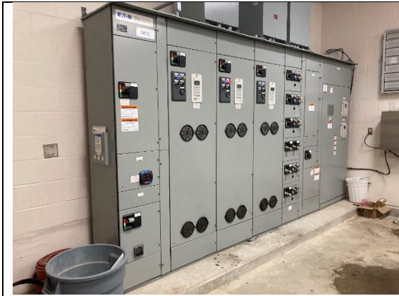
FIGURE 22 - INTERIOR OF BROWNLEY CHEMICAL STORAGE (NORTH-EAST) SITE
