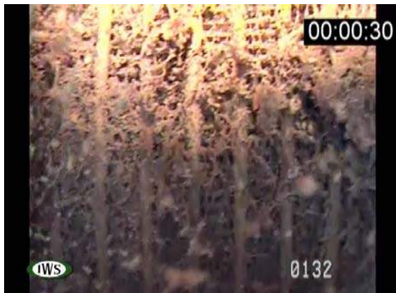
Horizontal view deposits on screen at 132 feet
