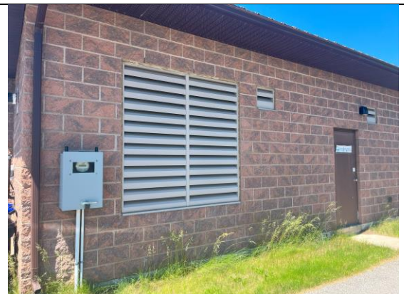
FIGURE 17 - EXTERIOR OF BROWNLEY CHEMICAL STORAGE (EAST) SITE
