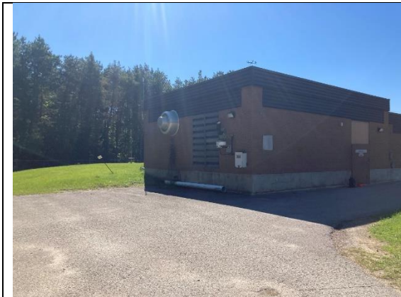
FIGURE 1 - EXTERIOR OF MILL STREET (NORTH-WEST) SITE
