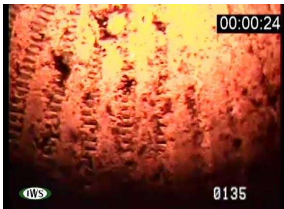
Horizontal view deposits on screen at 135 feet
