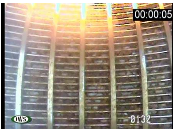
Filter pack material seen behind screen at 132 feet
