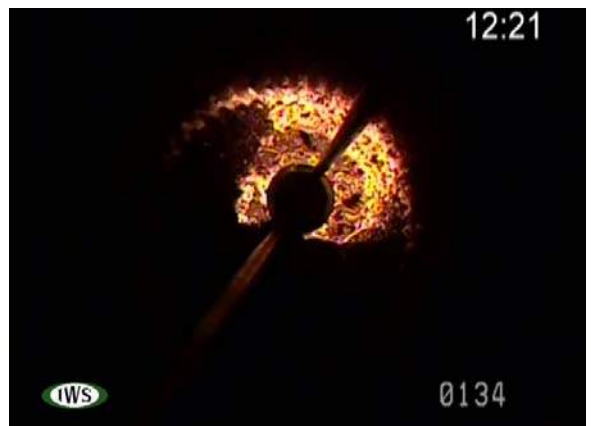
Partial blockage near bottom at 134 feet
