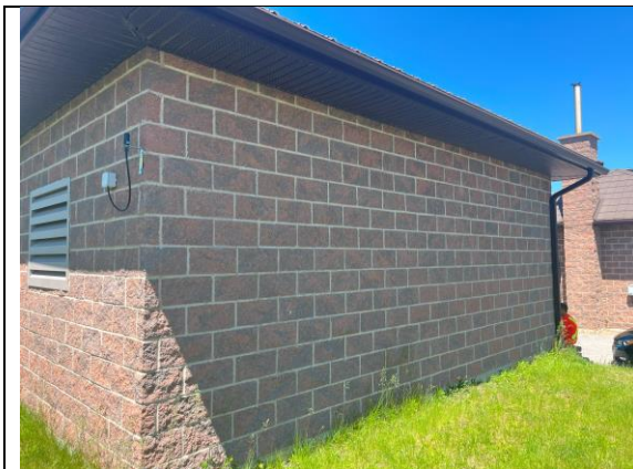
FIGURE 14 - EXTERIOR OF BROWNLEY PUMPHOUSE (EAST) SITE
