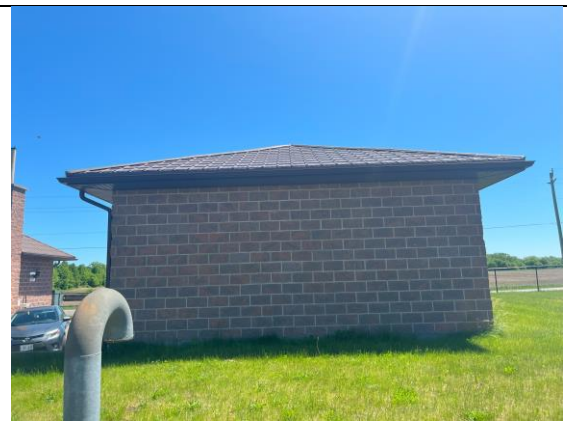
FIGURE 15 - EXTERIOR OF BROWNLEY PUMPHOUSE (WEST) SITE
