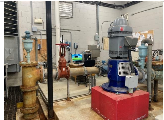
FIGURE 4 - INTERIOR OF EXISTING MILL STREET PUMPHOUSE (NORTH-EAST) SITE
