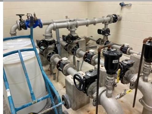
FIGURE 21 - INTERIOR OF BROWNLEY CHEMICAL STORAGE SITE
