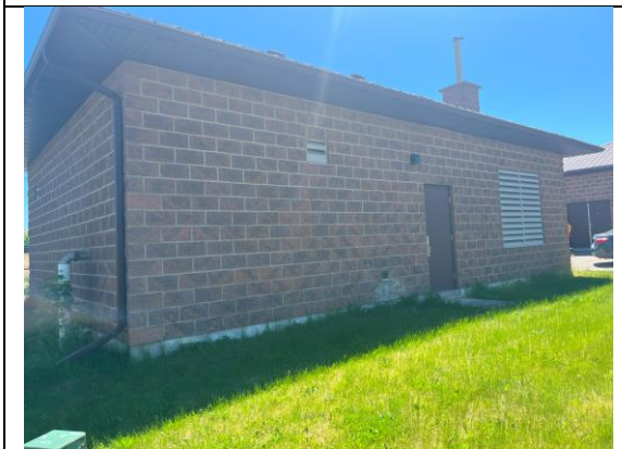
FIGURE 16 - EXTERIOR OF BROWNLEY CHEMICAL STORAGE (WEST) SITE
