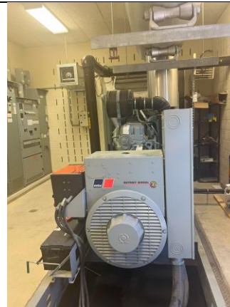
FIGURE 23 - INTERIOR OF BROWNLEY CHEMICAL STORAGE SITE
